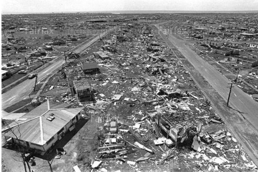
Figure 3. Housing damage in Darwin following Cyclone Tracy 1974 (credit: Fairfax Photos)
